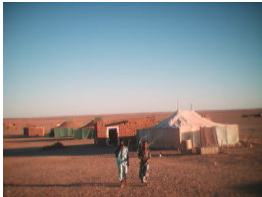
Smara photo caption: The outskirts of the Smara camp give a picture of typical construction within the camps. The tent and mud brick homes must withstand temperatures over 50° Celsius and ferocious sandstorms in what is commonly referred to as the "inhospitable Algerian desert."
